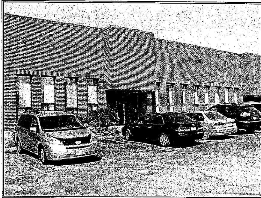
Front View of Subject Property
