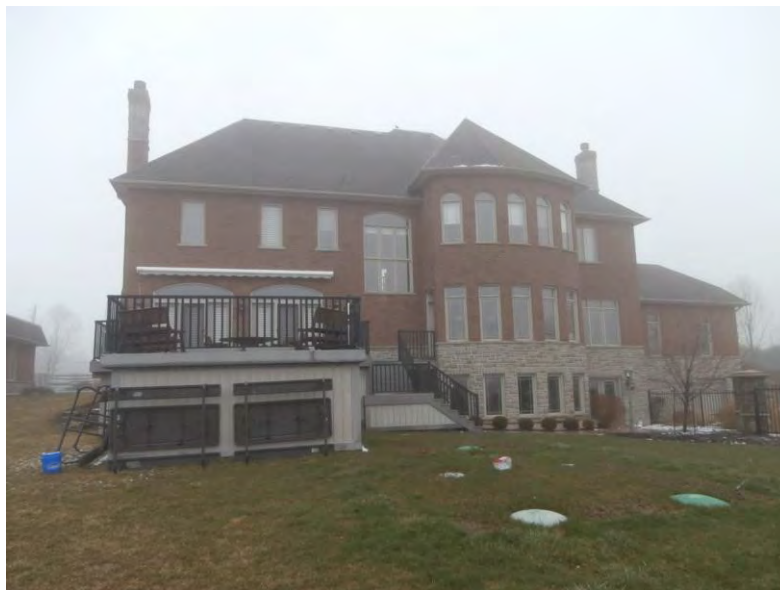
House Rear View (West Side)
